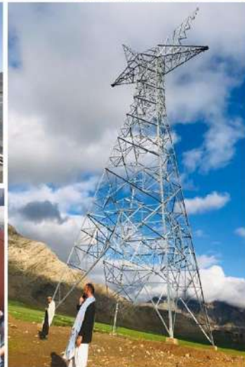
LOC. NO. : AP 1255 - EXCAVATION CASA 1000 200 KY AFGHANISTAN
