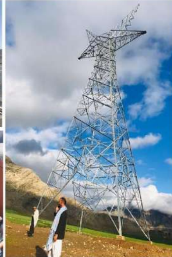
LOC. NO. : 1255- EXCAVATION CASA 1000 200 KY AFGHANISTAN
