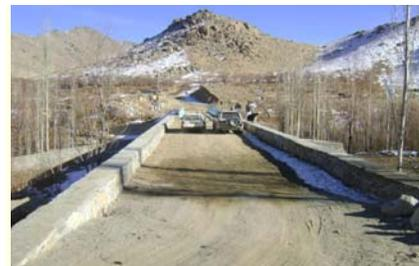
Construction of 58 m retaining wall and approach road in Hosa Bridge, Ghazni.
